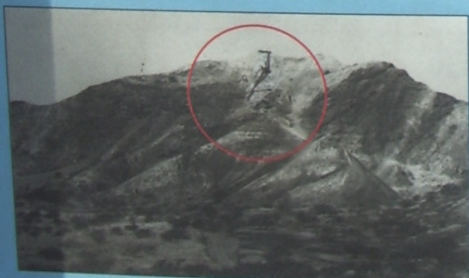
Construction of the trail and the Fire Control Station at the summit involved the removal of a portion of the crater rim. The excavated dirt was sent down a chute and deposited on the lower, interior slope of the crater.
