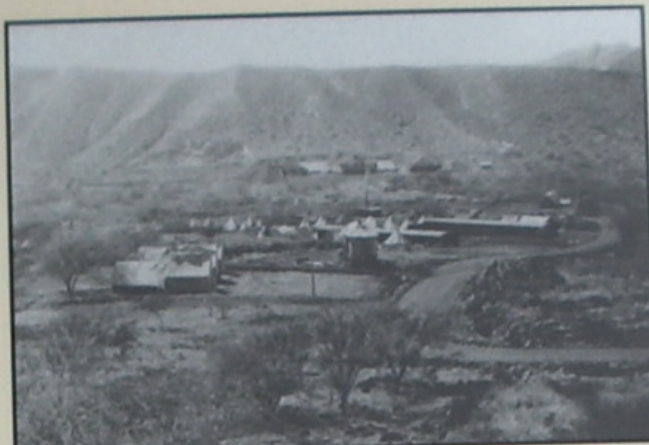
Constructing Fort Ruger and Battery Harlow on the outer, inland slopes of Diamond Head, circa 1908.
