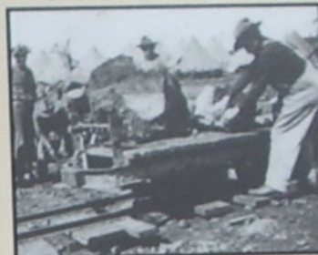
Small gauge railroad tracks were used to move rocks and supplies through the tunnels.
